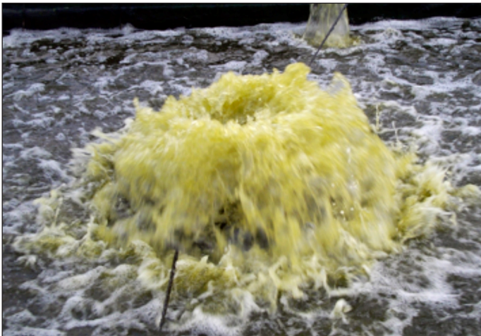
Figure 3: A surface aerator supplementing RAS aeration during peak loading in a green water tilapia system.
